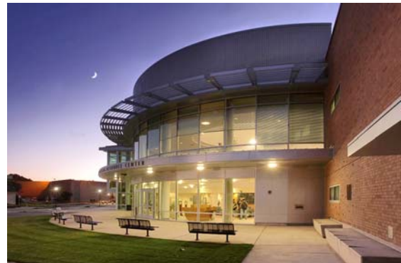
Hartnell College Learning Center, Salinas CA. Architect: BP Architecture, Concord, CA. Photograph ©2006 by Bob Swanson, www.swansonimages.com .
